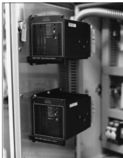
Drivers SMD15B mounted on the door of the control cabinet.
